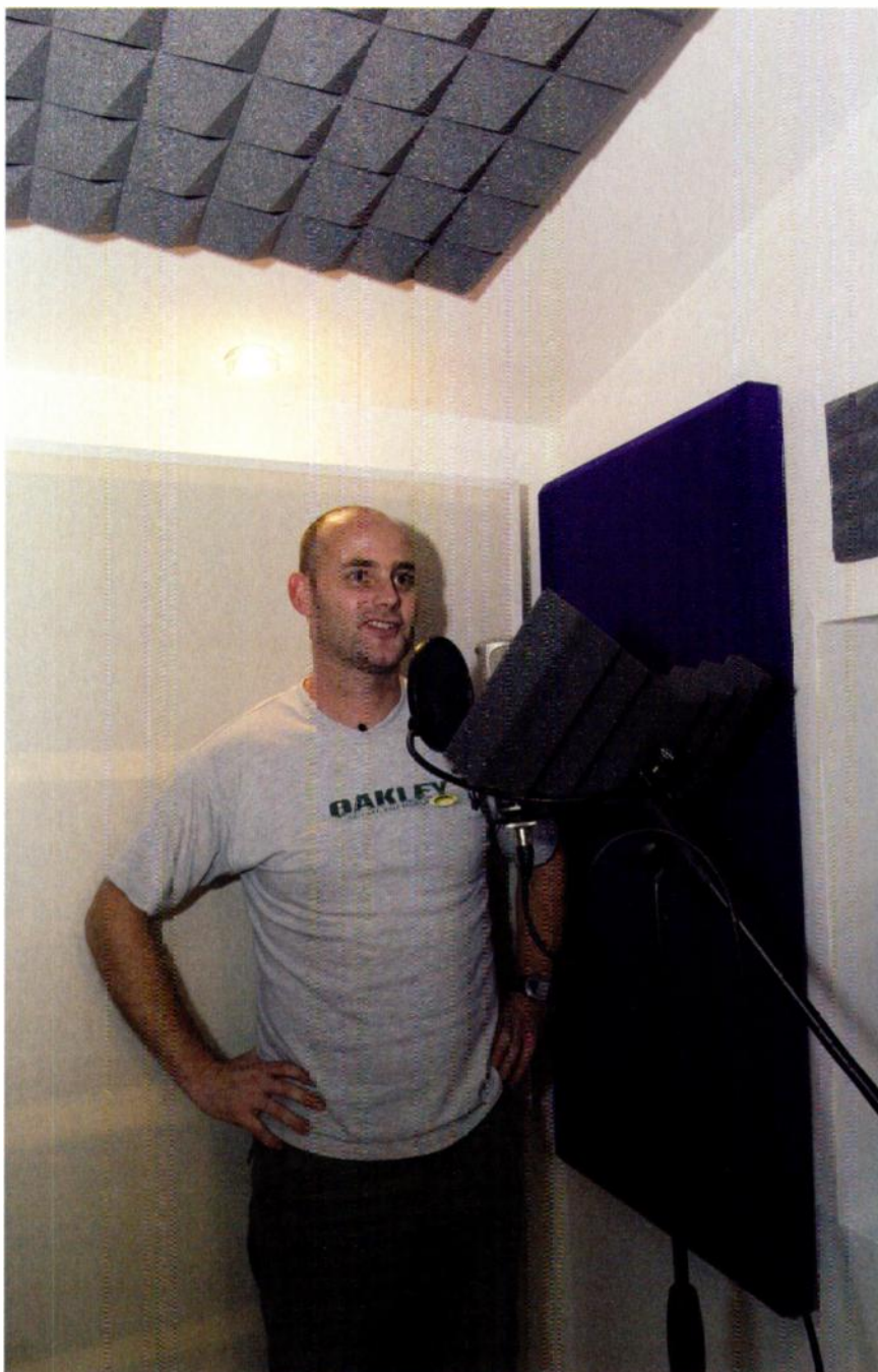
The finished vocal booth, complete with rear-wall bass trapping, side-wall and ceiling acoustic-foam treatment, and a 'butterfly' foam baffle fixed to the stand behind the mic.
