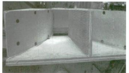
PHOTO 18: The completed throat reflector in place.
