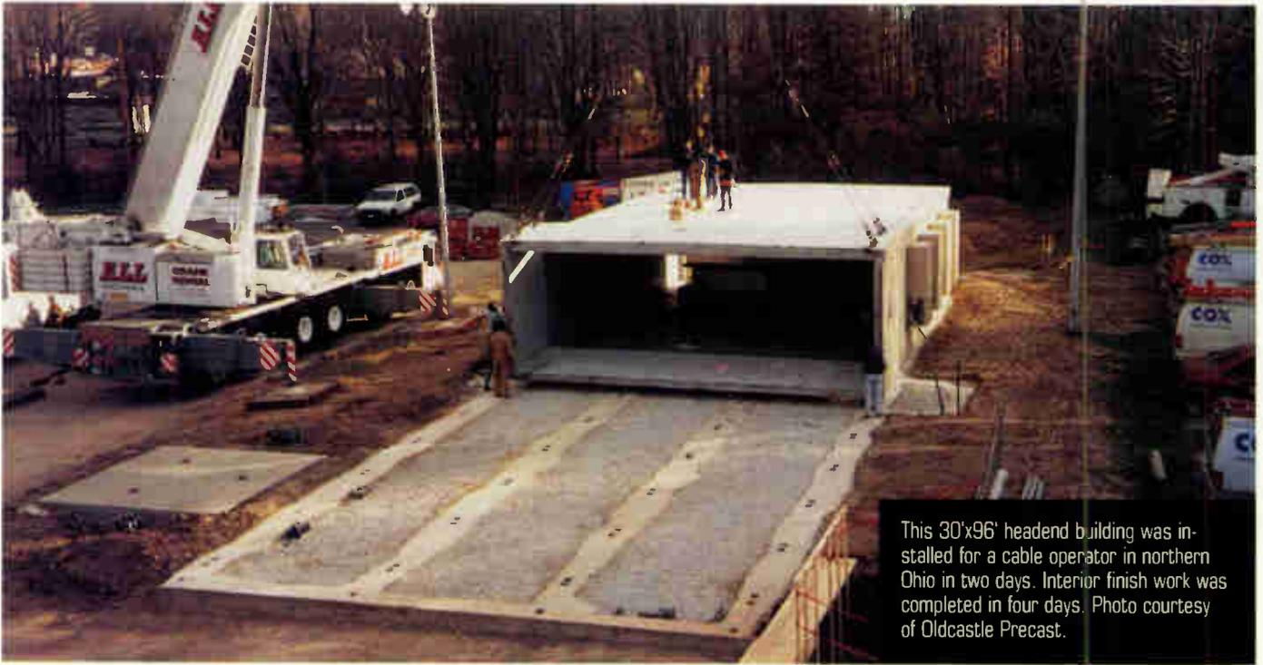
This 30'x96' headend building was installed for a cable operator in northern Ohio in two days. Interior finish work was completed in four days. Photo courtesy of Oldcastle Precast.
