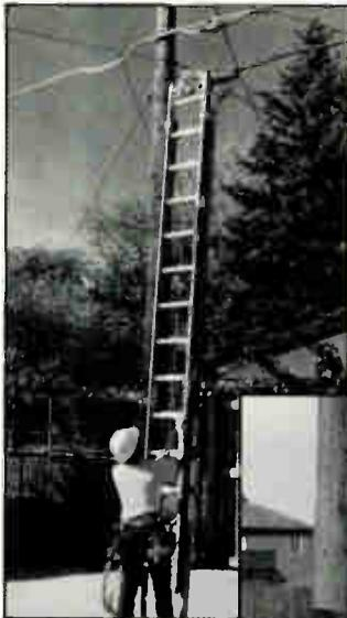
Proper safety gear is essential for pole-climbing and ladder work. Note the hardhats, eye protection, gloves, boots, safety harnesses and lanyards. Photos courtesy of NCTI
