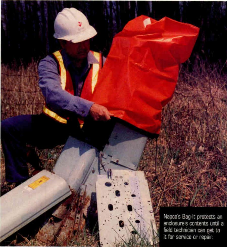
Napco's Bag-It protects an enclosure's contents until a field technician can get to it for service or repair.
