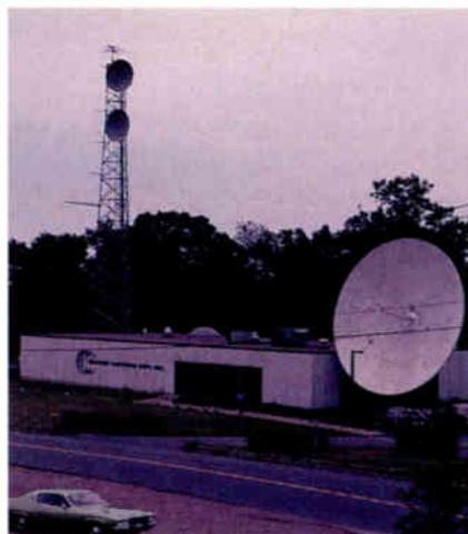
Greater Hartford Cable TV, August 1979: Notice the 10-meter antenna pointed at Satcom 1, the only satellite needed at the time.
