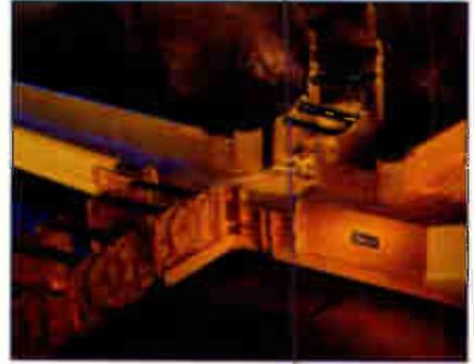
and provide protection from having coupling and mounting hardware on the outside of troughs.
