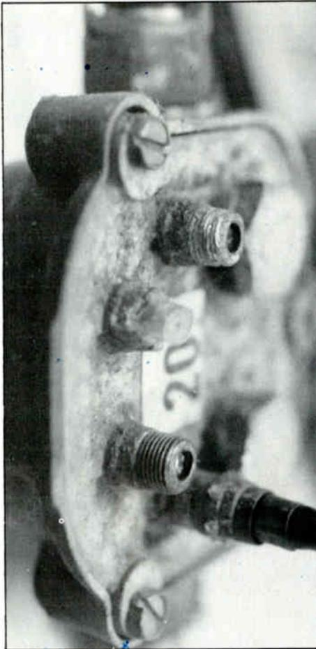
**Corroded tap fittings prevent good ground contact while broken fittings prevent installation of terminators.**
