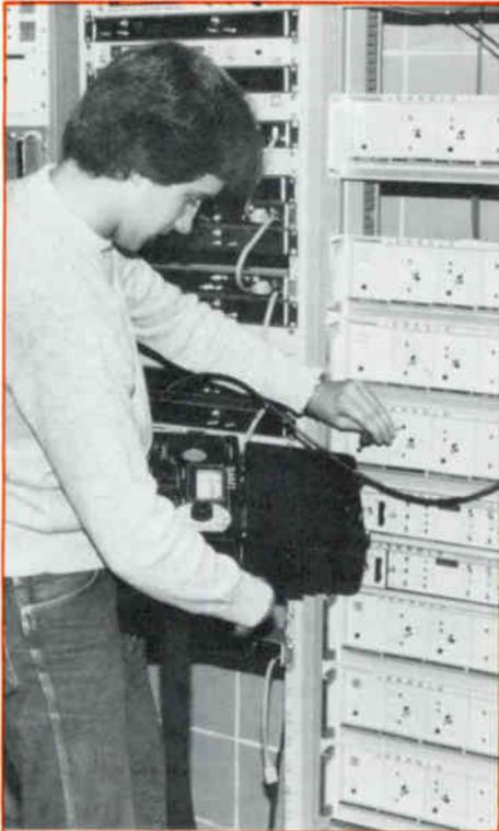
*A student adjusting a processor in the school's headend, using a signal level meter. Because this headend serves only the school he can take as much time as is needed to do the job right.*
