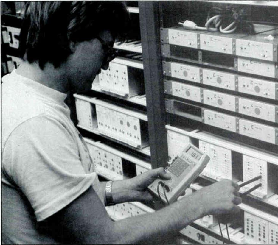
**Caltec Headend Technician Tony Kern measuring AGC voltage on a fiberoptic receiver. This reading corresponds directly to the optical power of the incoming signal. This test, along with others, are conducted every three weeks as part of the preventive maintenance program.**
