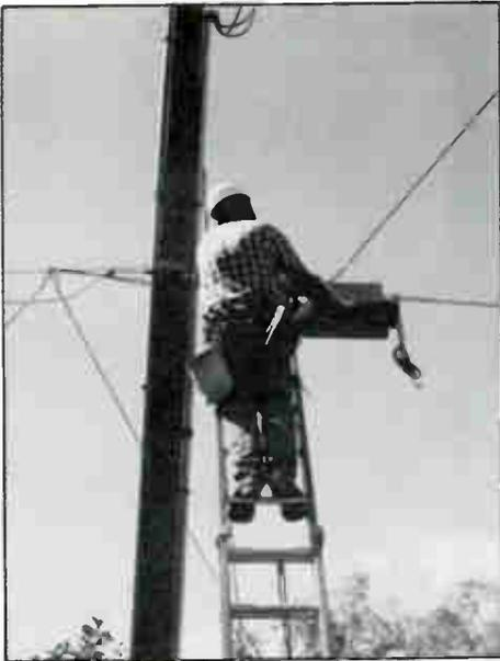
**OTAS strand-mounted terminal being installed.**
