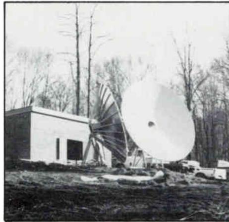
**The satellite antenna placed near protected, low ground for good reception.**
