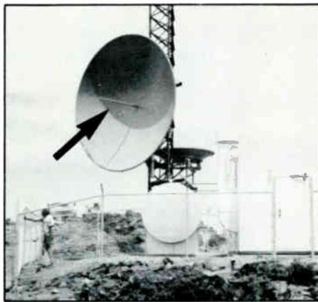
**A typical microwave antenna (note the arrow pointing to the feedhorn).**
