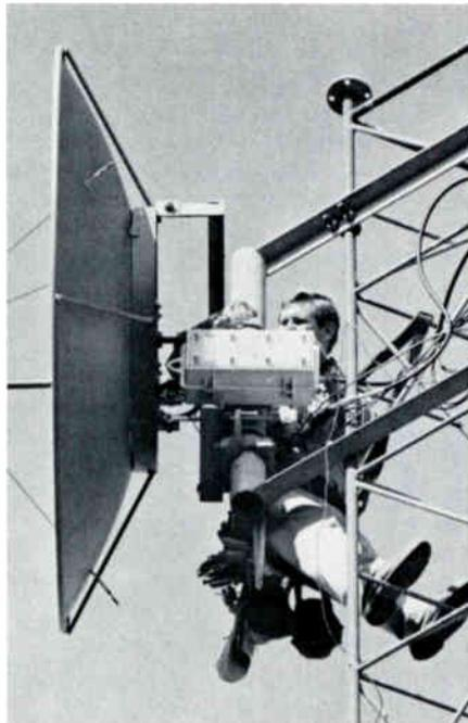
In addition to extra power, the 5-watt system utilizes GaAs FET amplification, highly stable microwave oscillator and redundancy of key components to insure reliable operation and reduce maintenance. A Status Monitor Panel, included with the 5-watt transmitter, allows remote monitoring of all system functions by bringing all test points to the headend or tower base.
