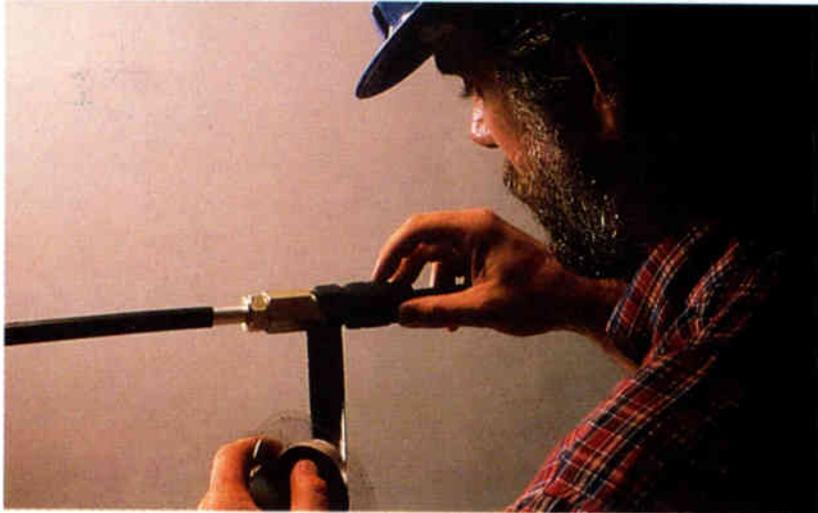
Take the easy, one-step method to seal out moisture and to corrosion protect your CATV equipment. Raychem's GelTek™ sealant strip will wrap around, adhere instantly and conform to the many sizes and shapes found in your system. Even irregular connectors like right angle and housing to housings can now be protected.
