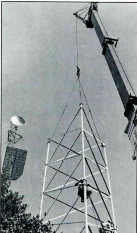
**Clockwise from above: self-supporting tower being erected using a crane; pier-and-pad foundation for guyed tower base under construction; foundation reinforcements for "dead-man" anchor block for guyed tower.**
