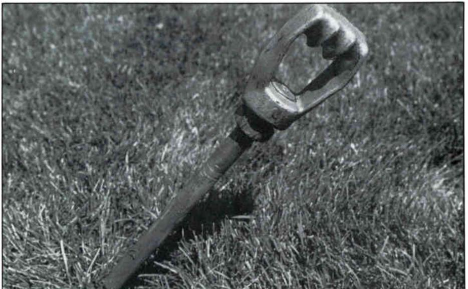
*After the load locker is removed, the thimble is screwed onto the end of the anchor rod, ready for guying.*
