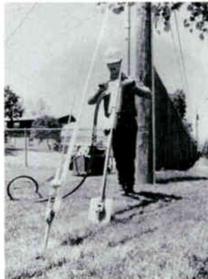
*One man at ground level drives Manta Ray with jack hammer.*
