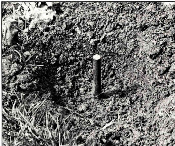
*Photo 1: Drive the ground rod into the ground using a suitable sleeve or driver so the top of the rod does not mushroom.*
