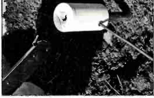
**Photo 8:** Ignite the starting material with the flint ignitor, holding it one or two inches from the hole in the mold cover.
