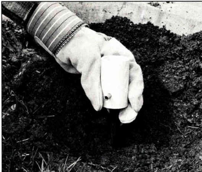
*Photo 2: Install the mold on the rod being careful not to damage the rubber gasket on the bottom of the mold.*
