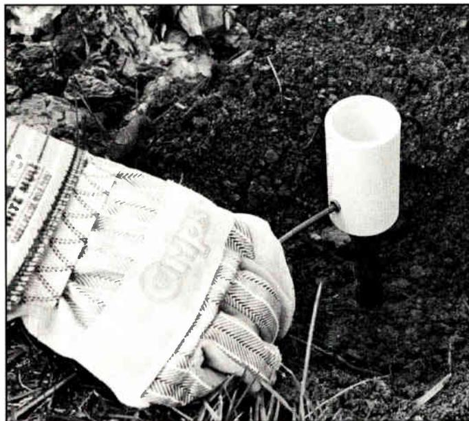
*Photo 3: Insert the ground wire through the sleeved hole in the side of the mold until the end of the wire touches the opposite inside surface of the mold. Push down on the mold until the top of the ground rod comes into contact with the bottom of the sleeve and ground wire.*
