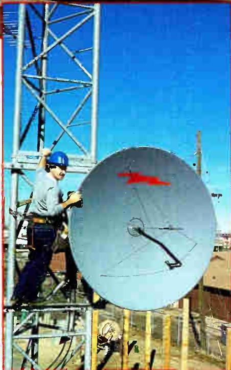
*Aligning the microwave path.*
