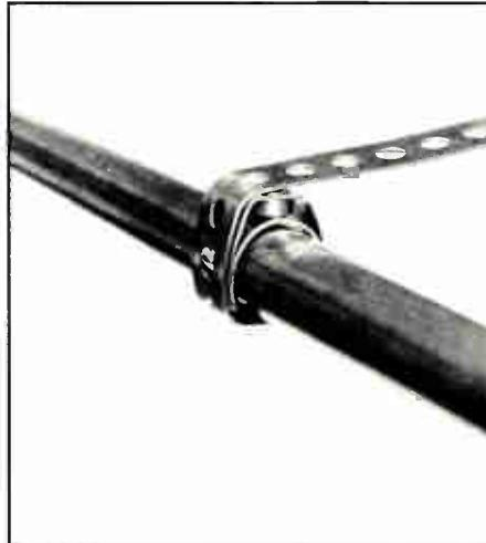
**Step 5:** Fold the strap over itself snugly until the second hole above the alignment tab lines up with the threaded hole for the bolt.
