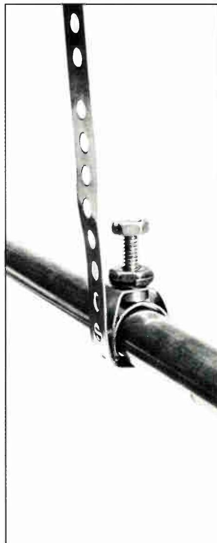
**Step 3:** Wrap the strap tightly around the pipe, then line up one of the holes with the strap's alignment tab. This will temporarily hold the strap in place. Do not tighten the strap at this point (that will stretch the strap or break off the tab).
