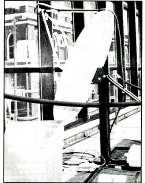
**Channel Master and Viacom Nashville installed a microwave link to provide local signals to the exhibit area.**
