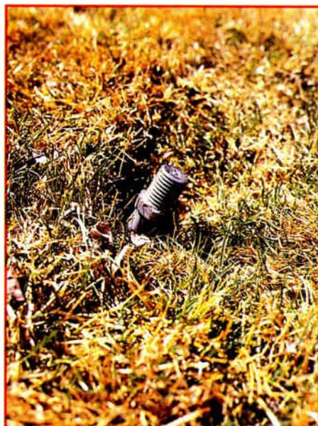
**Photo 4:** End of anchor rod is at ground level.
