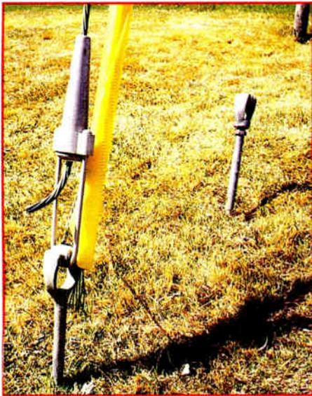
**Photo 7:** After Load Locker is removed, thimble is screwed onto end of anchor rod, ready for guying.
