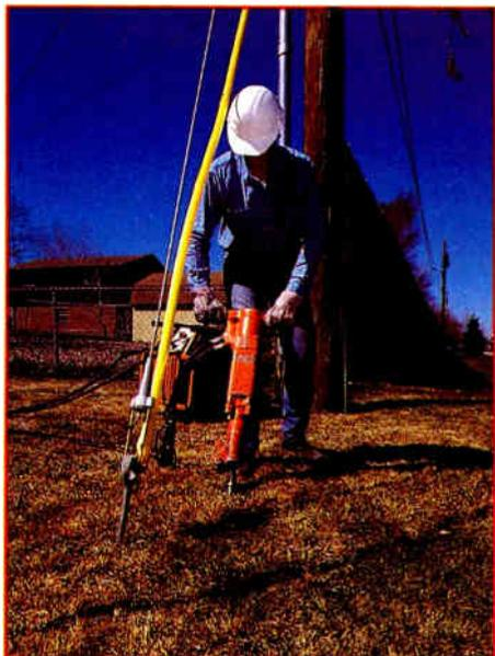
**Photo 2:** The anchor is now at the desired depth.
