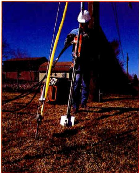
**Photo 1:** Installer starts anchor into ground.
