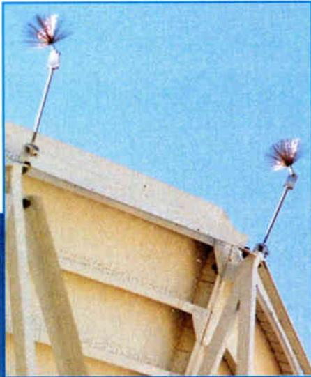
**Metal satellite dishes can be protected by installing a dissipator array directly on the frame at the top.**
