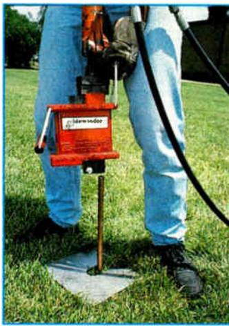
**Photo 9: Steps 6 through 8 are repeated as necessary until about 1 foot of the rod remains above the ground. The Sidewinder is then placed on top of the rod for the final step.**
