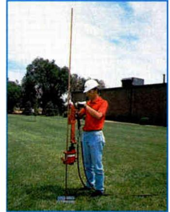
**Photo 4:** The entire assembly is lifted to a comfortable driving position, and the installation process begins.
