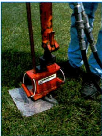
**Photo 5:** The ground rod is driven into the soil until the Sidewinder reaches ground level and contacts the release plate.
