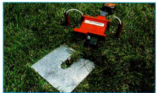
**Photo 10: The ground rod is driven to the desired depth.**
