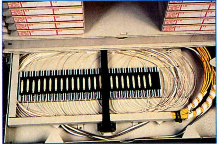
Keep the splice trays covered and sealed to protect fiber ends and avoid excess moisture, which may degrade the fiber's mechanical and handling characteristics.
