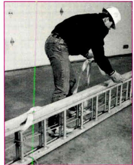
**5) Secure the other end of the Ladder Tote to the ladder rail three rungs from the center position in the opposite direction.**
