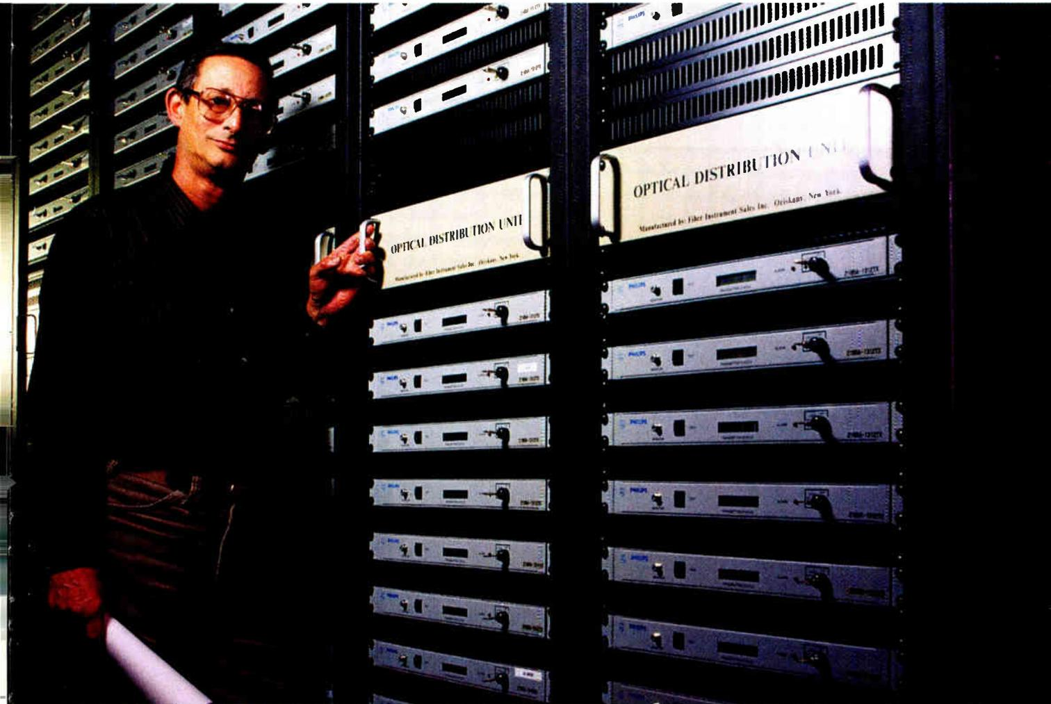
“Every quarter we test our fiber optic COAX system and compare current trace signatures to the originals to spot problems before our subs view them. We’re shooting Laser Precision’s mainframe and Mini-OTDRs, which let us pinpoint faults, too.
