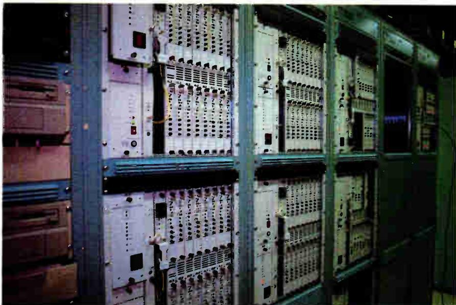
*MediaOne's ADC DB6000 digital video equipment, that is used to digitize the video signal up to 16 channels each for distribution to remote hubs.*
