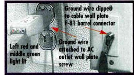
Figure 2: Temporarily grounding ungrounded polarized two-slot receptacle
