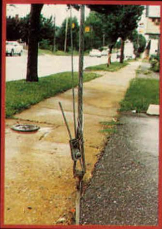
Top left: The CATV system is just a few inches from street light power. Top right: The NEC does not permit grounding to a flexible conduit. Bottom left: A missing down guy guard presents a hazard to pedestrians. Bottom center: The
