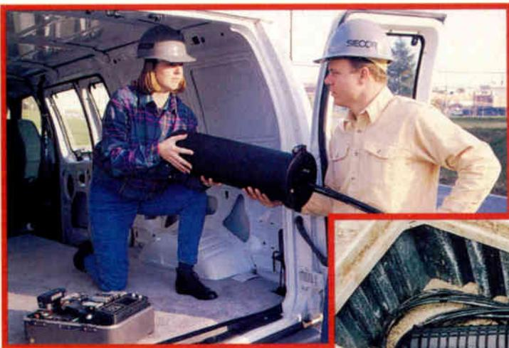
Enclosures protect your fiber splices from water ingress. Placing them in vaults enables re-entry.
