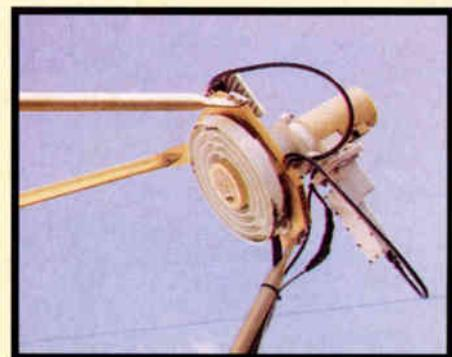
Even a small hole as seen in the lower part of this feedhorn screen can cause maintenance headaches. Carefully inspect the entire satellite dish for damage.
