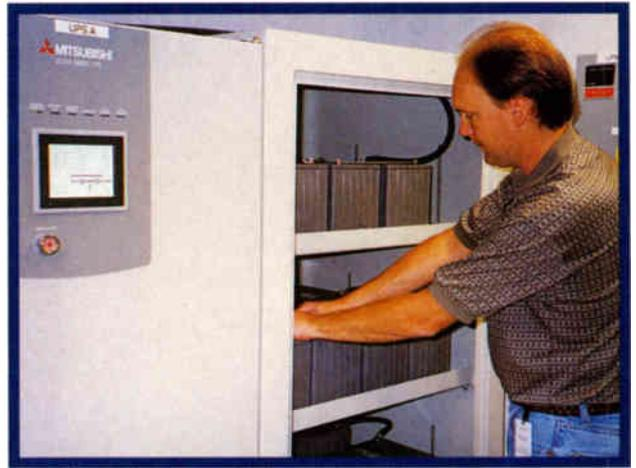
Battery-powered universal power supplies, such as this 50 kW unit, provide temporary electricity to Cable TV Montgomery's headend until the onsite generator turns on.
