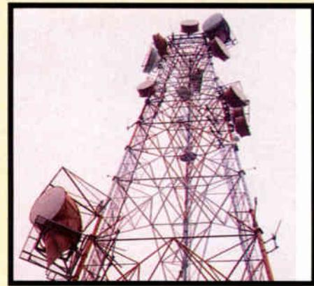
Tower inspection includes checking feedhorn covers and ice shields, not to mention the antenna mounts.
