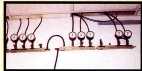
A nitrogen manifold not only gives an individual level of pressure for each line, but the individual line valves permit quick isolation of any leaks.
