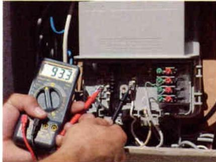
Above: A technician verifies 90 V of power at the NIU. Right: An installer inserts a PCT pin into a power-passing tap, using a plastic sleeve to prevent shock. Photos courtesy of Cox Communications, Orange County, Calif.
