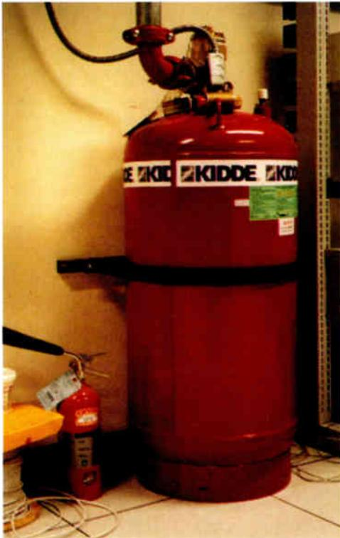
Fire suppression, such as this FM200 system in Cable TV Montgomery's headend, becomes increasingly important as headends deliver a complex mix of must-have digital services.
