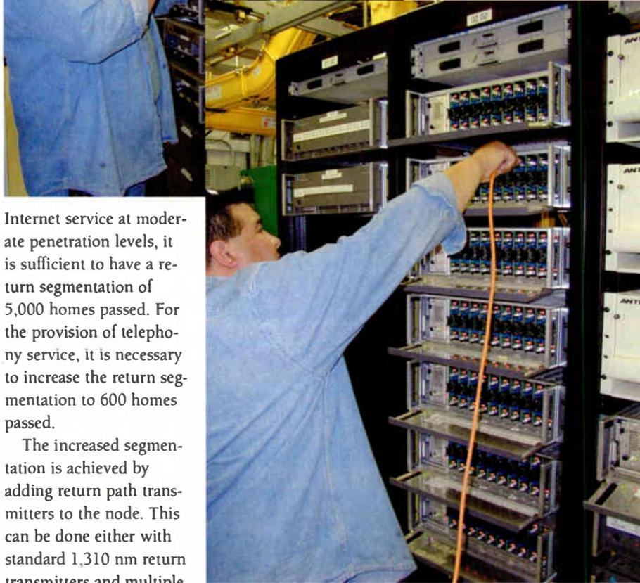
Internet service at moderate penetration levels, it is sufficient to have a return segmentation of 5,000 homes passed. For the provision of telephony service, it is necessary to increase the return segmentation to 600 homes passed.
