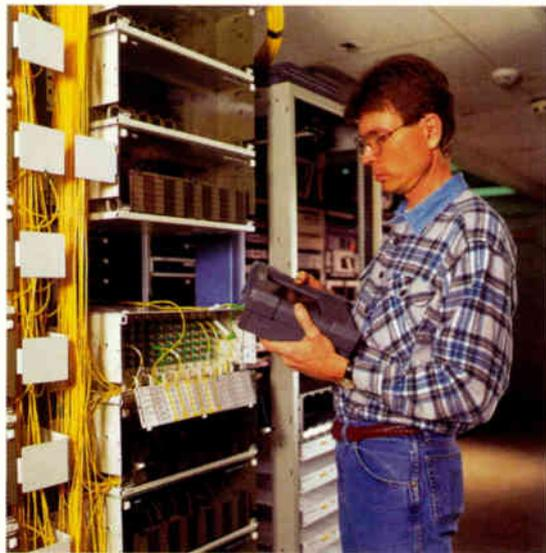
Using an OTDR with a high dynamic range can help you speed the time it takes to get a good trace.
