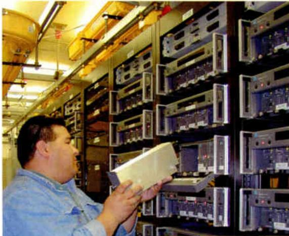
In another look at the AT&T B&IS Aurora system, at left, a technician mounts a narrowcast forward path transmitter module. Below, the tech tests the RF signal level on a return path receiver. Both photos courtesy of Harmonic Inc.
