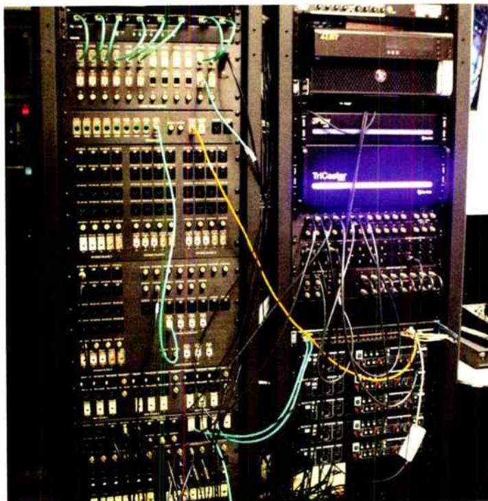
The wiring rack is the central nervous system of the entire facility. This rack includes KVM switches and Cisco switches for the AoIP network, as well as the TV production equipment and PEG channel server.
