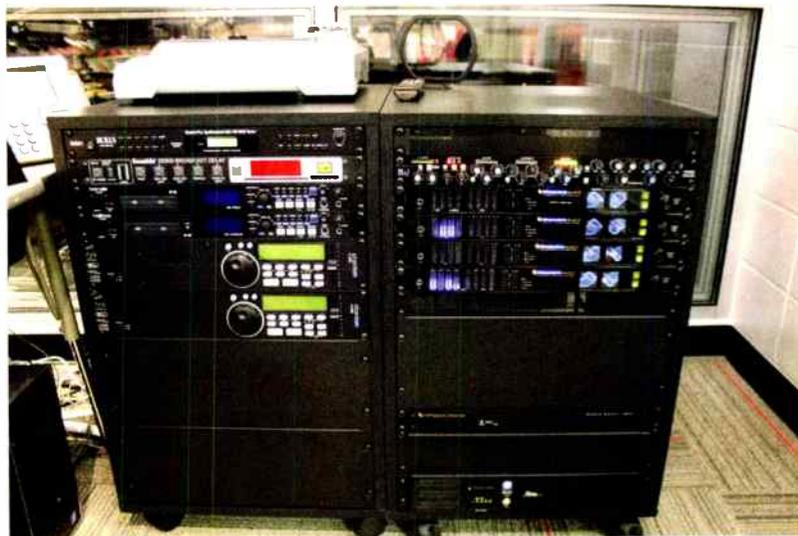
Each radio studio has identical racks. The racks were intentionally made to be shorter in order to maintain sightlines.
