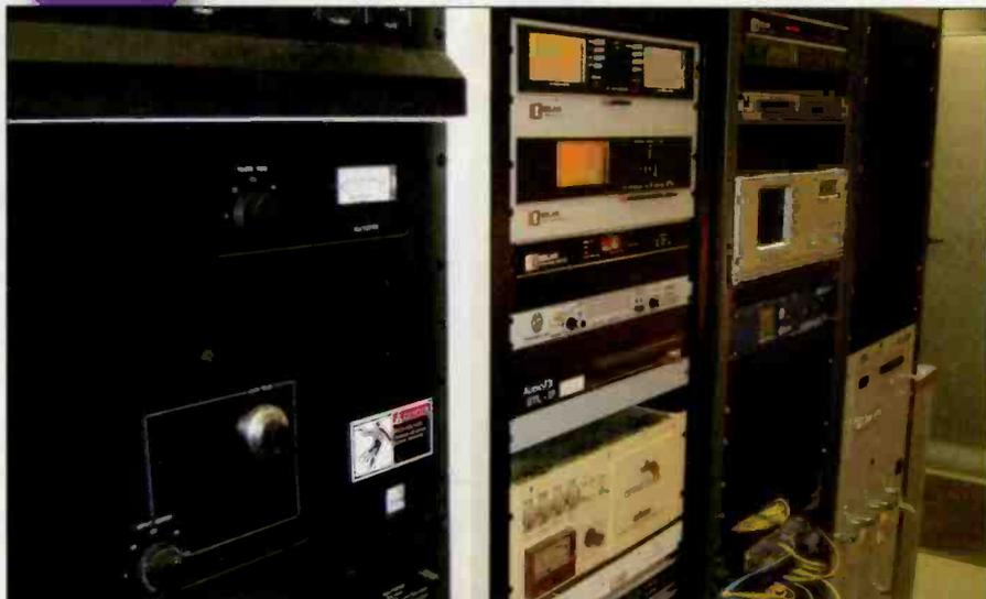
Repeater station WKRW has the 1992 installed analog Harris transmitter and the new IBOC transmission equipment behind.
