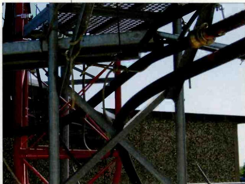
**The lower transmission line is loosely resting on the metal braces, which will likely wear a hole in the outer jacket.**
