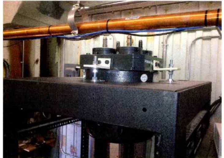
Figure 3: Four-Port Switch Mounted in the Top of the Equipment Rack
