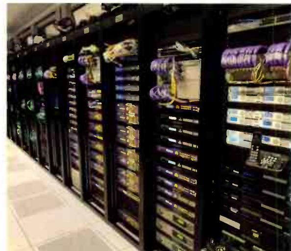
Banks of audio codecs and audio routing hardware in the tech core.
