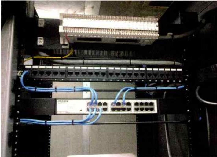
Figure 2: Network Switch, Patch Bay and Krone Block
