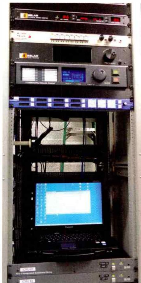
Although disconnected from the studio, the network at the transmitter continued to work, allowing the Burk Plus to function normally. Operators could dial into the Burk Plus for readings and control.
