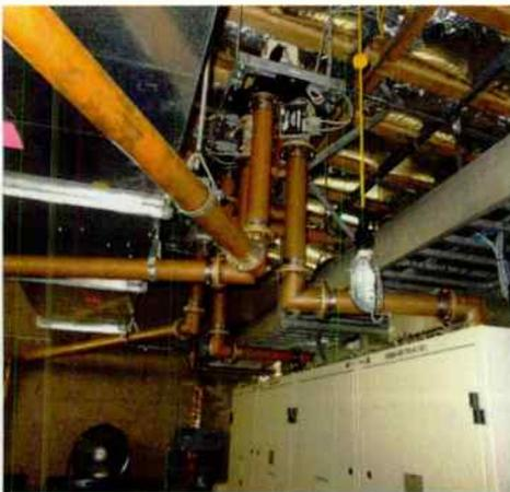
Coaxial switch and transmission line routing for KCBS-FM and KTWV transmitters
