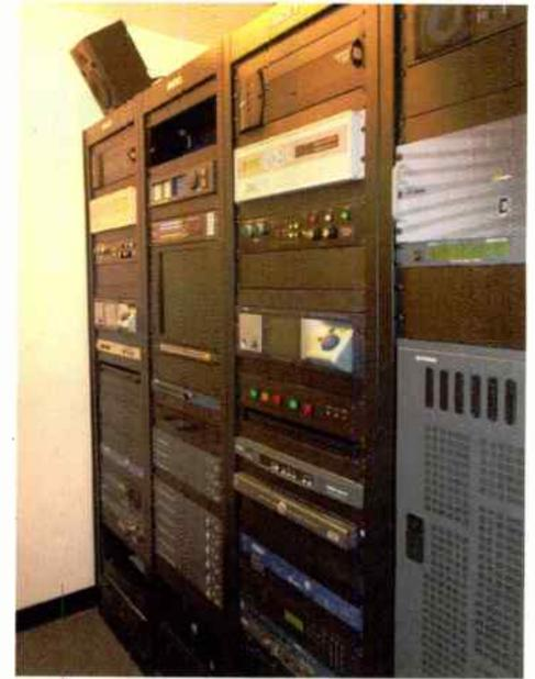
Racks at the Verdugo bunker site, including the KAMP auxiliary transmitter, a GatesAir ZX-5000
