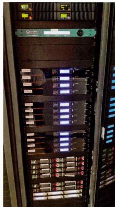
A stack of DaySequerra monitoring receivers in the technical operations center.
