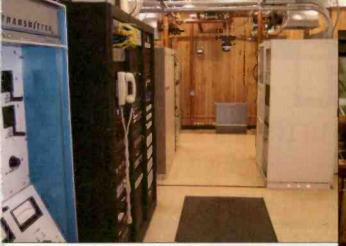
Flagship station WKSU's analog equipment row on the left and its Harris Z model IBOC transmitter on the right across from a Broadcast Electronics FM-20T analog transmitter installed in 1997.
