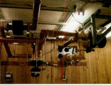
A close up view of WKSU's split level 1BOC combining system and main/standby antenna switch.
