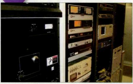
Repeater station WKRW has the 1992 installed analog Harris transmitter and the new IBOC transmission equipment behind.
