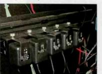
plug-strip from BSW. This plug strip has metal brackets that are adjustable for various size wall-warts and allows them to be securely clamped in place. The cord is grounded and heavy-duty and the mounting holes permit several mounting configurations. He chose to mount his on the side-rails of the Middle Atlantic rack at the transmitter site.
