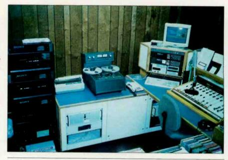
The on-air combo studio for country-formatted WOHT-FM and WDTL-FM in Cleveland, MS, uses a Computer Concepts DCS (monitor at upper right, controlling hard-disk spot storage) with a TM Century UDS (controlling Sony CD jukeboxes at left). Each station uses the studio for separate live or live-assist dayparts. During dayparts when both stations are fully automated (mid days and overnights), the studio is used for production.
