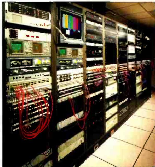
Atlantic Satellite is linked by 50 digital fiber lines to Waterfront facilities, and the uplink service utilizes Waterfront for delivery of video. Atlantic Satellite's satellite receiver rack is shown here.
