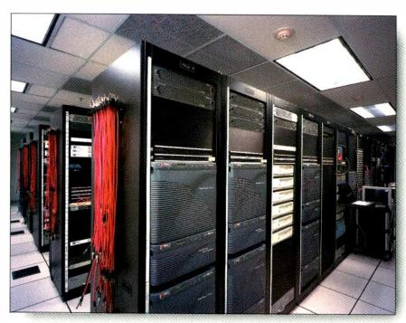
Pinnacle redundant video servers in the central equipment room are shown above, with the A server (air) on top and the B (backup) on the bottom of each rack.
