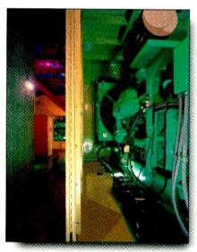
The facility utilizes redundant 750kW generators to guard against system failure.
