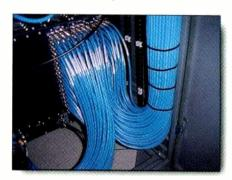
The rear of this small router shows smooth cable radius and good cable support.
