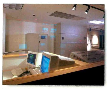
Smart System Controller Computer displays (nearest computer) are used for monitoring HVAC performance and individual rack temperatures. The farthest monitor displays parameters for redundant UPS, power distribution units and generators.
