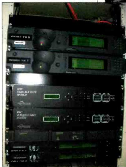
and performance on the old link. MRC helped develop a link budget and, based on the numbers, suggested 16 QAM as the level to ensure acceptable performance during worst-case conditions. The maximum bit rate on the link is 60Mb/s with the 16 QAM modulation spread over three IF channels in the variable rate modem.
