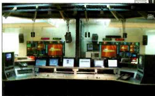
This area provides operators with a final look at a signal before it leaves the building. A Snell & Wilcox RollCall network monitoring and control system is instrumental to this room. The facility's main RollCall terminal is installed here to monitor equipment and pinpoint signal loss quickly. With 500 racks throughout the facility, the system minimizes failure effects.
