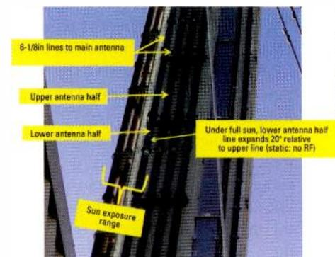
Figure 11. Transmission line configuration on tower
