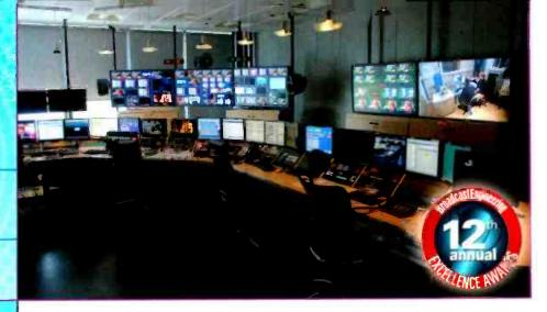
o guarantee the durability of its activities in Europe, the cultural channel Arte has adapted its site to HD. Arte has also decided to transfer the entire workflow of the company to a file-based environment by adopting the AVC-I@100Mb/s MXF OP1b-wrapped format.
