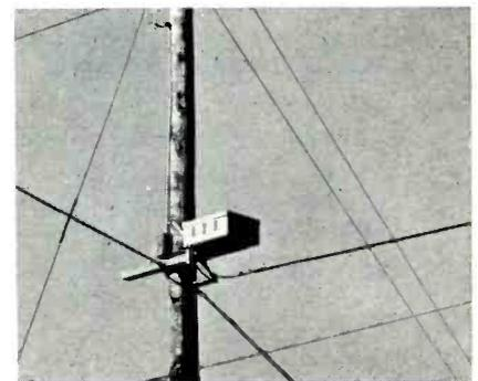
Fig. 5. Amplifier in protective enclosure.
