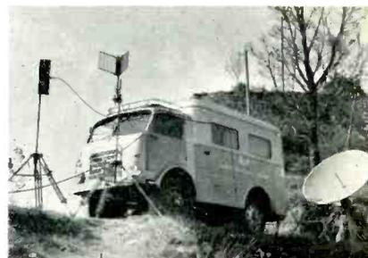
Fig. 3. Multiple-antenna ground station.
