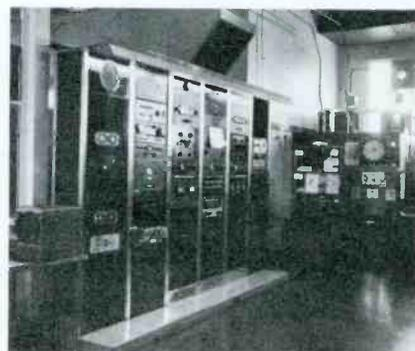
Audio and monitoring equipment now in use with the 50-kw transmitter is contained in these racks.
