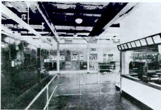
This view shows the WLW transmitter building as seen from the front entrance. The 50-kw exciter appears at the left, the 500-kw amplifier-modulator is in the background, and the audio control room is at the right. Circa 1934.
