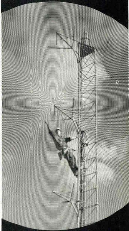
JAMPRO advanced technology has developed another industry "first"! A circularly polarized FM Antenna with variable horizontal to vertical gain ratios! Jampro will adjust the ratio to your exacting specifications for the best possible reception performance available—Reception to the outer fringes, and to more auto FM receivers, too.
