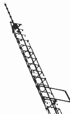
Omnidirectional transmitting antenna is side mounted with UHF unit on top.
