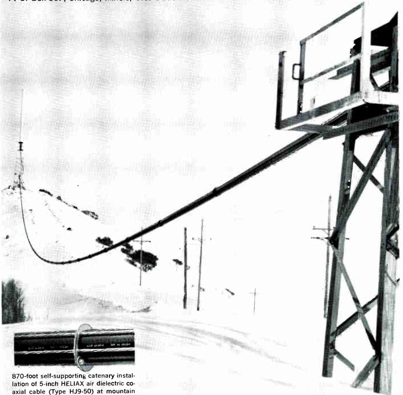
870-foot self-supporting catenary installation of 5-inch HELIAX air dielectric coaxial cable (Type HJ9-50) at mountain top site of Station KBYU-TV, Provo, Utah.
