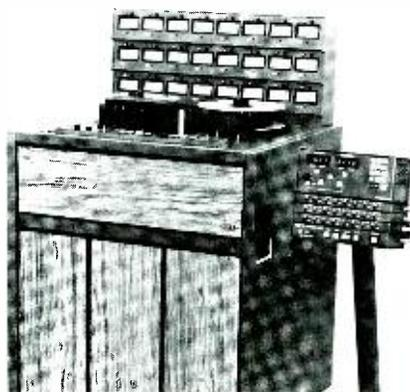
The JH-24 series of multi-track recorders is available in 8-, 16- and 24-track versions. Features include totally transformerless circuitry, quick-change tape format capability, full remote provided as standard equipment and the optional AutoLocator III, including 10 programmable memories, tape velocity indicator and yo-yo (repeat) functions.
